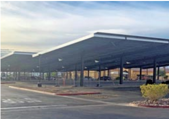
Solar panels structures at Mountain View Clubhouse parking lot
